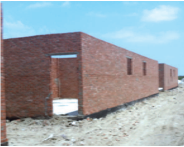
Figure 47. Government built recycling workshops in Port Said.
