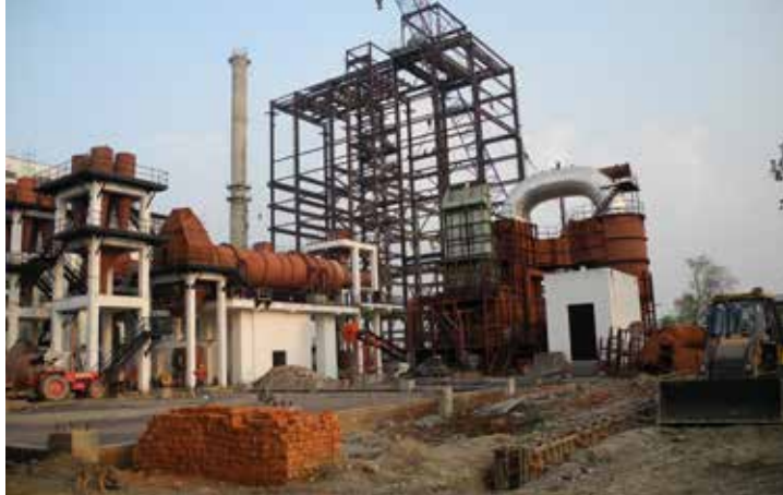
A cement plant under construction.
